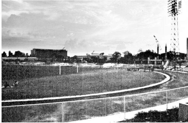
Chandrasekharan Nair Stadium gallery at the beginning of the construction, 1985
