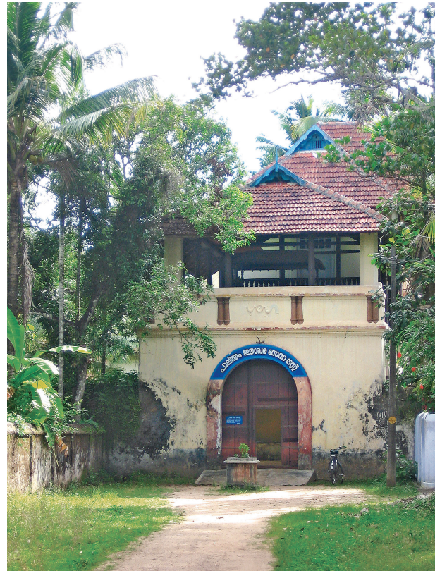
Paliyam Palace exterior before conservation
